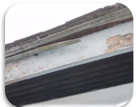
Rotten wood on this garage's fascia makes it relatively easy for animals to gnaw through. Repair or cover these areas with mesh to keep animals out
